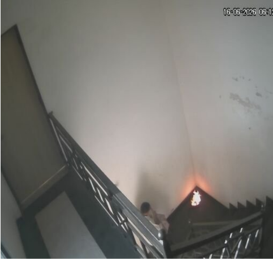
Staircase CONTROLLED DEMO
